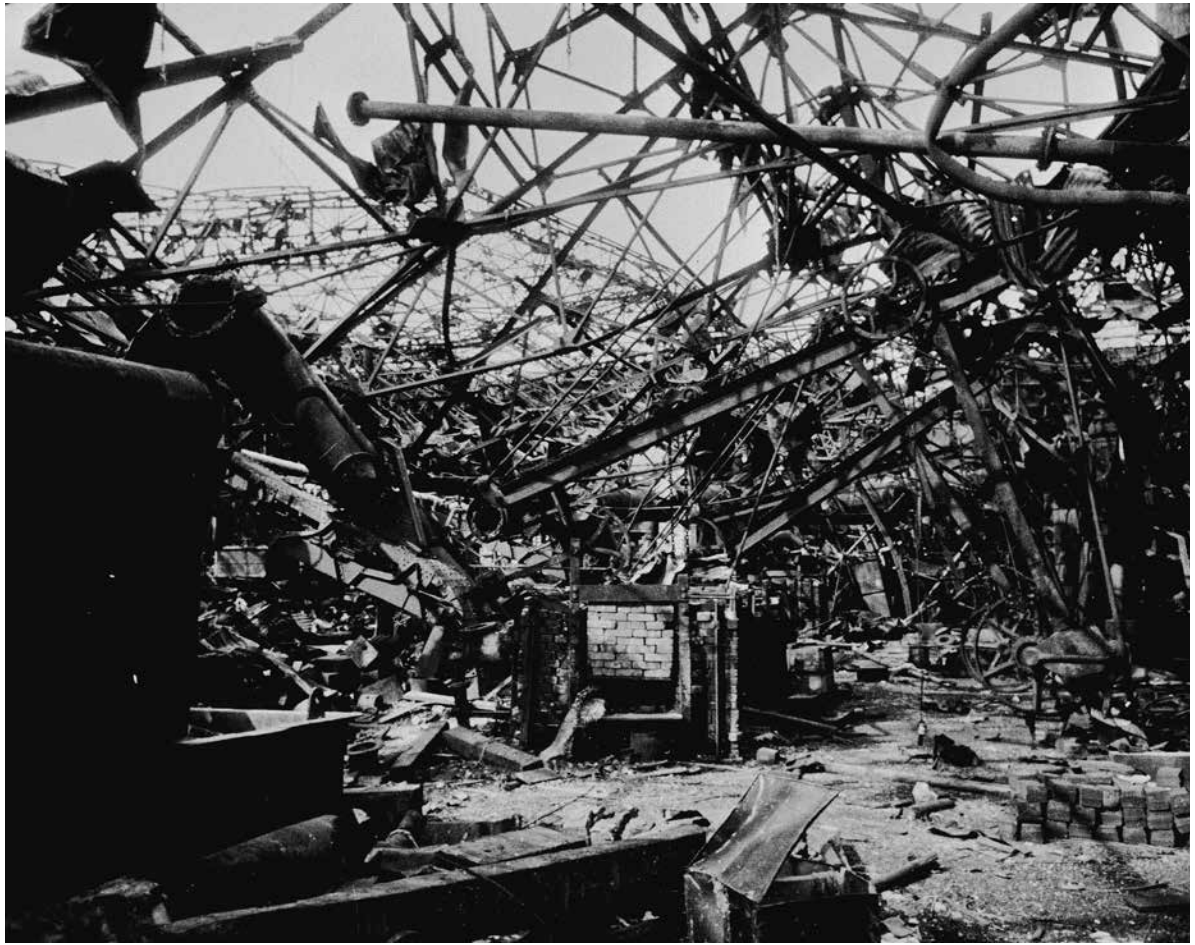
Flash of Light, Wall of Fire: Damage inside the Mitsubishi Nagasaki Steel Works No. 2 Plant, mid-October 1945 (Shigeo Hayashi).
